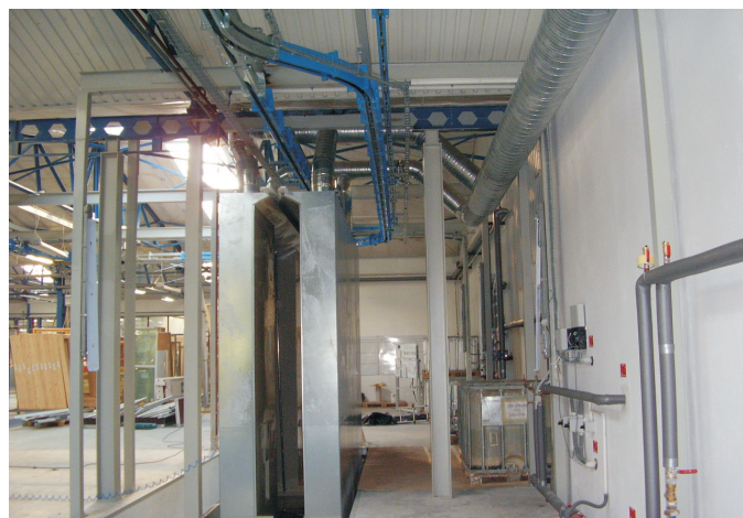
Flow-coat placeret i grav
